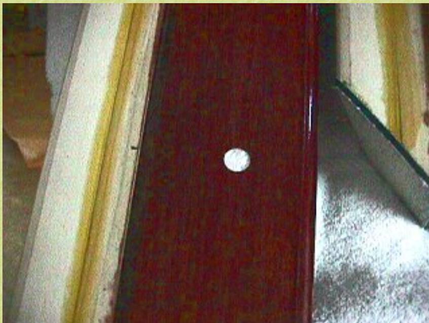
tight to go into the rail. Put some tightbond in the hole and use a flat block of wood to tap the sight into the rail so that it is flush. Wipe off the excess tightbond with a damp cloth and shine it up with a dry cloth. This will ensure that there is not glue residue on the rail.
